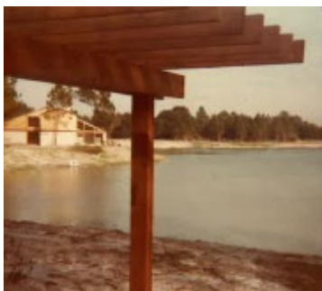
Construction on the Big Lake
